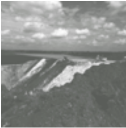
Inert earth stacking at Moissy-Cramayel, 2019
